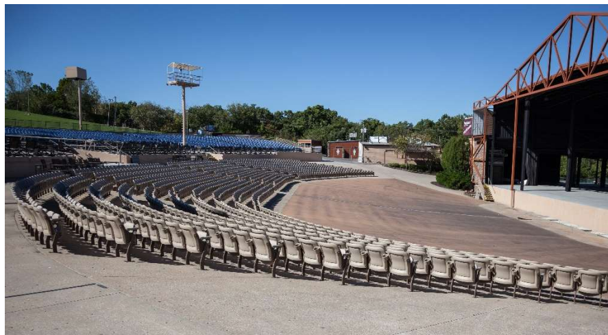
Open GA lower pit
